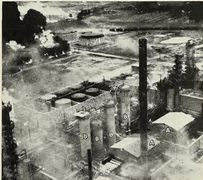
With storage tanks ablaze in background, bombers pass over cracking unit furnaces (A) and fractionating columns (B).
